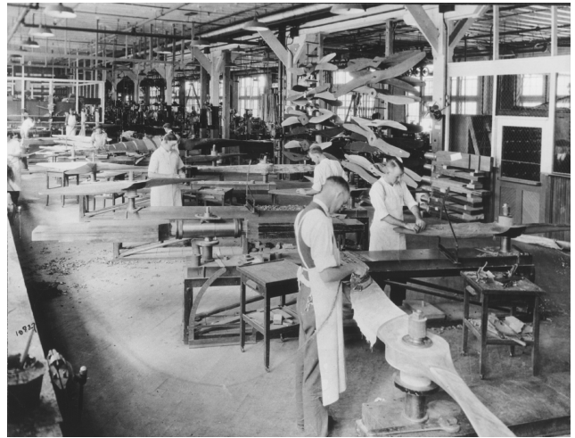
Craftsmen made wooden propellers in the McCook Field Propeller Shop.
