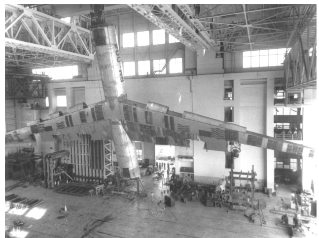
Fuselage and wing of the XB-36 being turned upside down for structural tests in the Static Test Facility, Building 65. (Bob Cavanagh)
